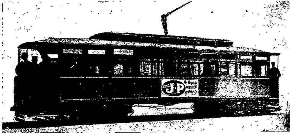
DOUBLE-BOGIE CAR BUILT BY THE BRUSH ELECTRICAL ENGINEERING CO.
